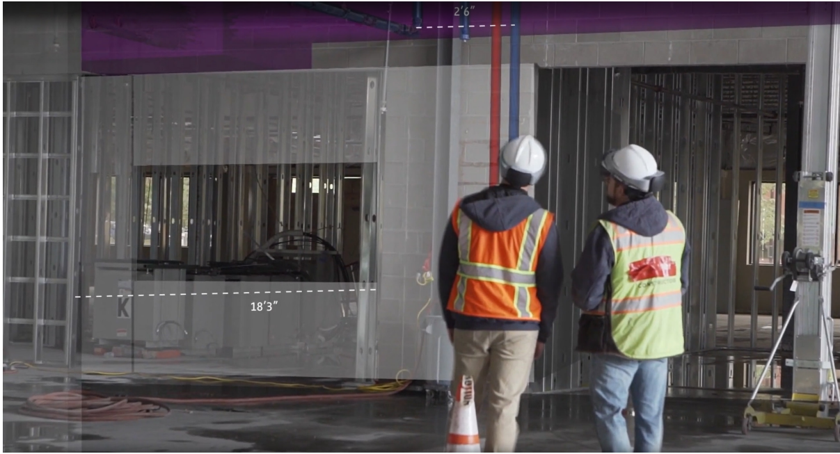
Figure 5 – Trimble Connect allows users to collaboratively view and interact with digital models whilst on site (Trimble, 2022).
